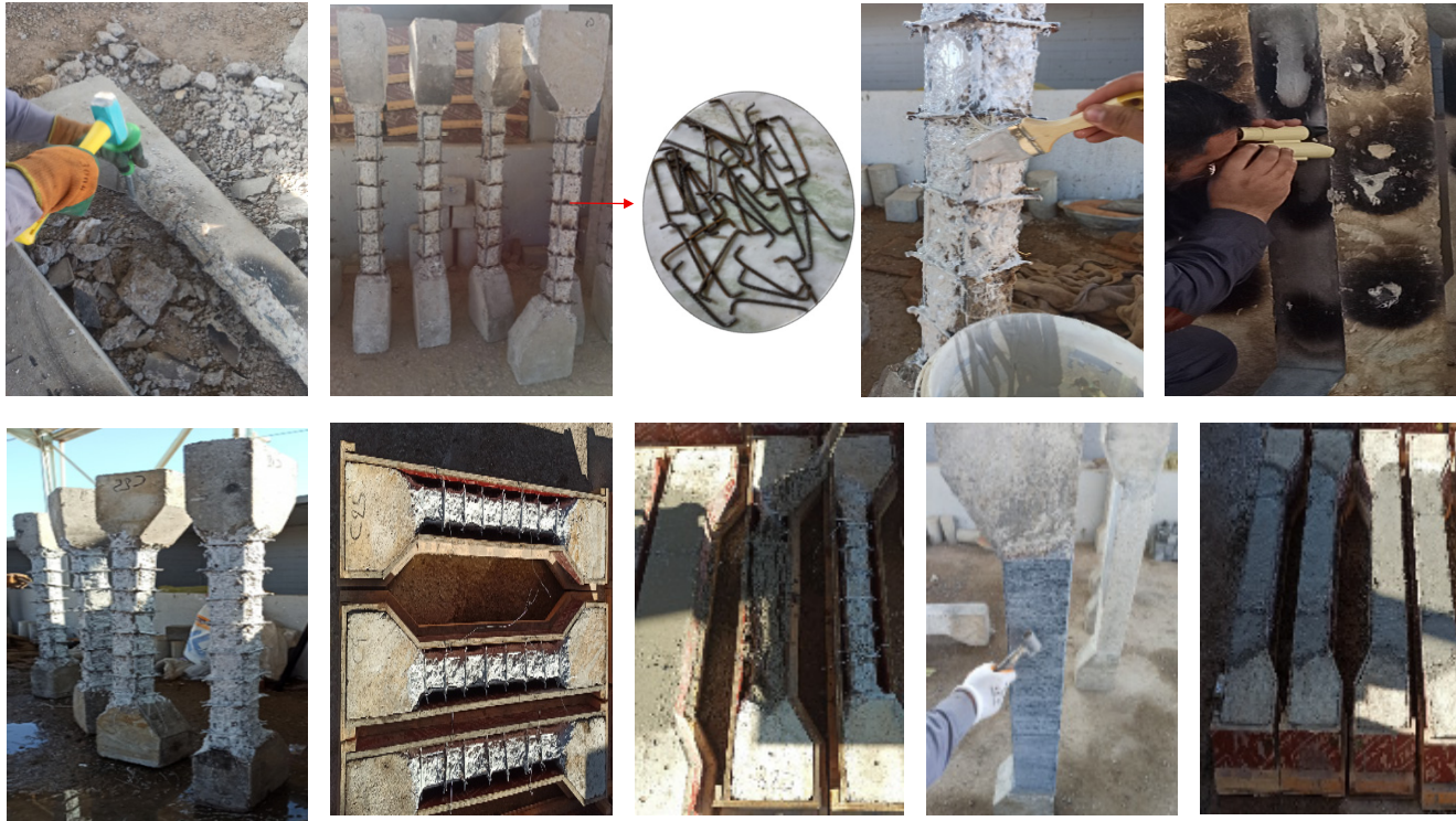
Fig. (6). Sequential steps of RC column repair.
